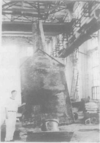
Fig.4 ESRC guide vane of hydraulic turbine for Three Gorges project
